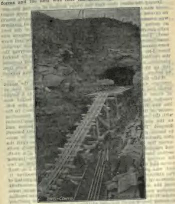
Fig. 5.—Method of Handling Concrete for Lining.
